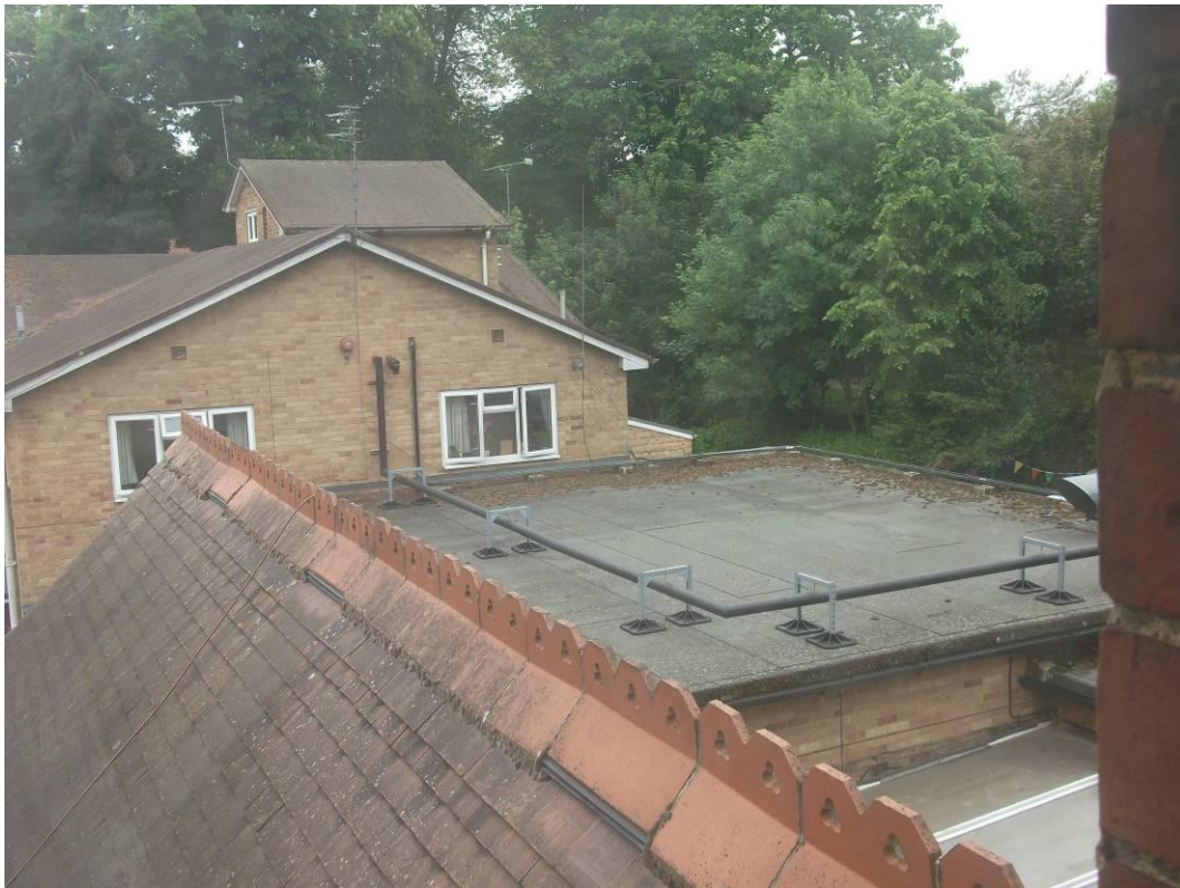
Photograph 14 (Kitchen / dining room roof)
