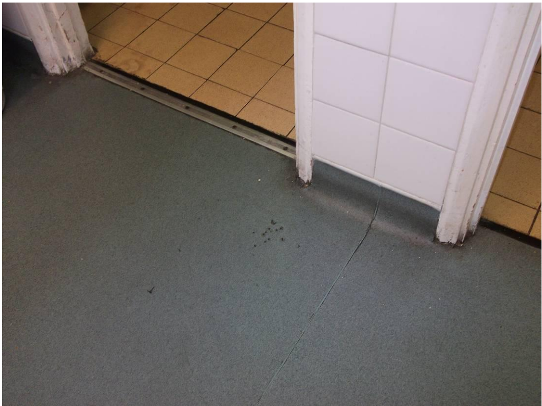
Photograph 34 (Kitchen vinyl flooring)
