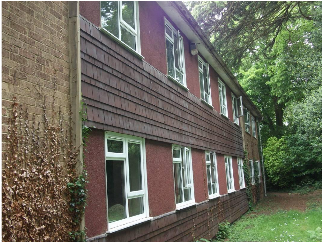
Photograph 09 (West elevation West wing)
