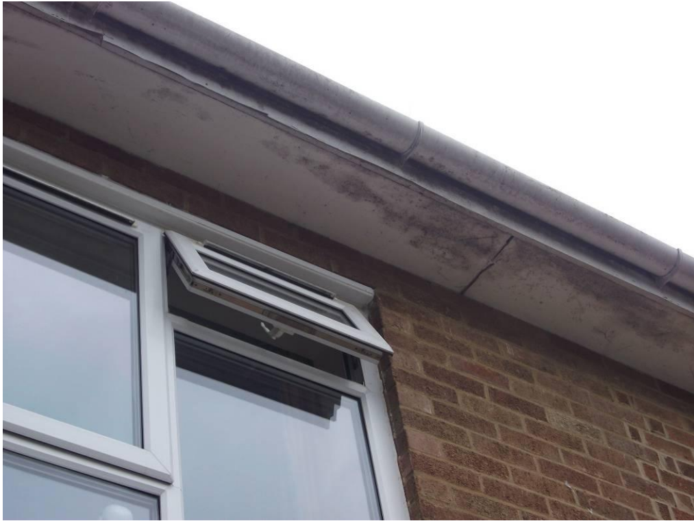
Photograph 05 (Soffit and fascia West wing)
