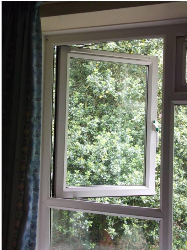
Photograph 18 (Typical bedroom window)
