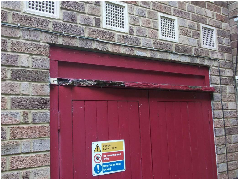
Photograph 08 (Boiler room doors)
