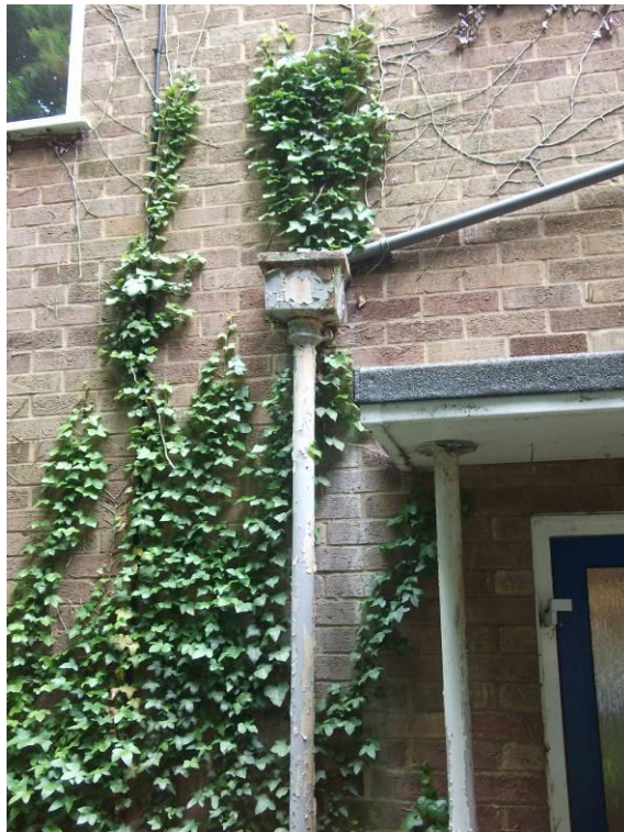
Photograph 06 (Drainage South elevation)
