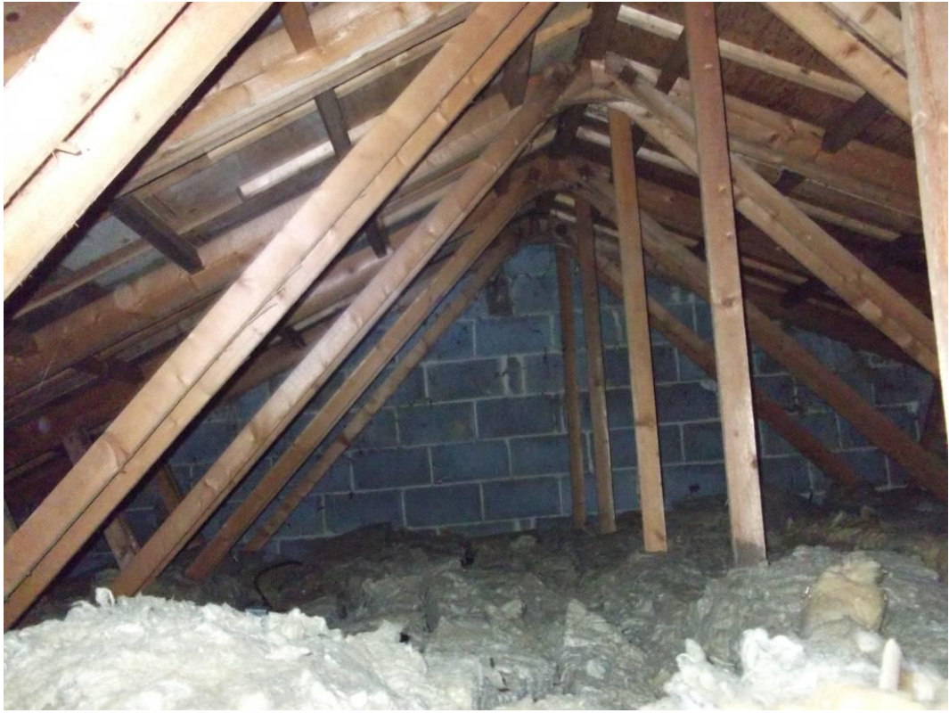
Photograph 27 (roof void West wing)
