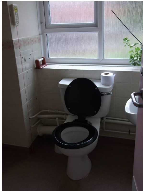
Photograph 22 (Typical WC adjacent bedrooms)
