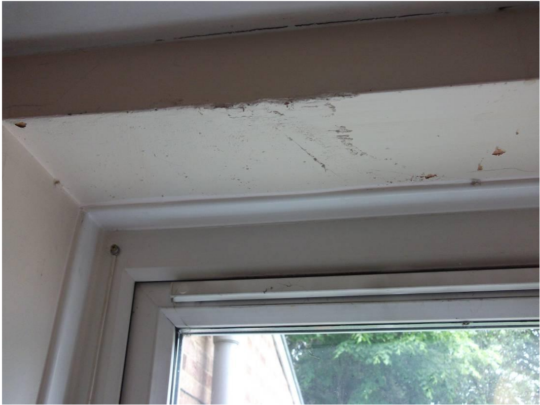
Photograph 35 (Head of window Kitchen)
