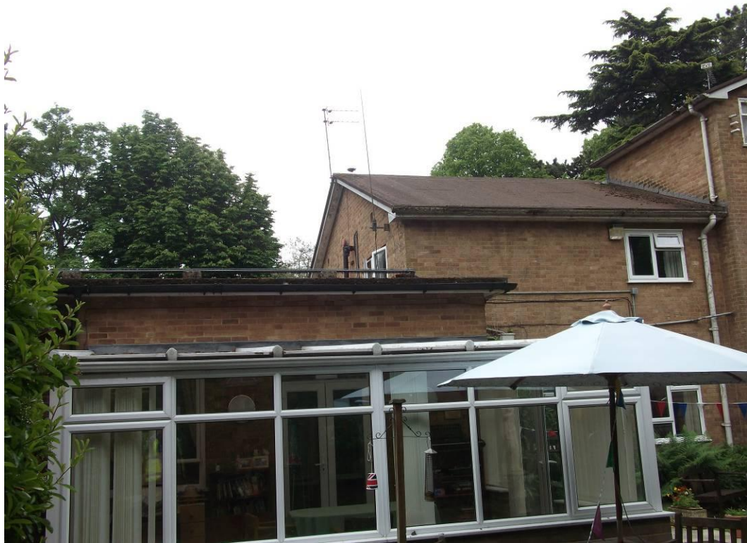
Photograph 10 (Conservatory of dining room West elevation)
