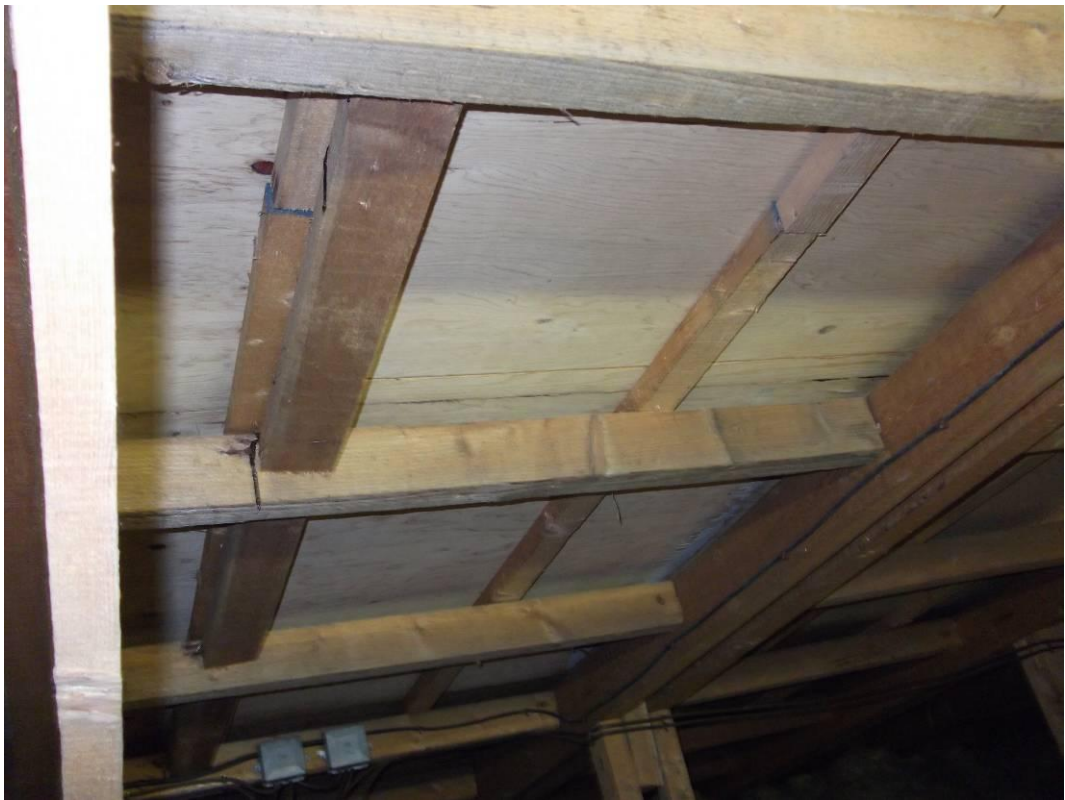
Photograph 28 (Typical roof construction)
