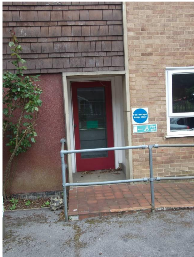
Photograph 04 (Fire escape West wing)
