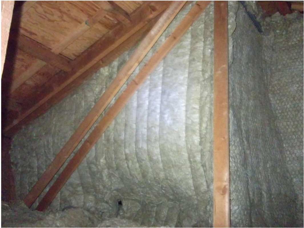
Photograph 29 (Fire break in roof void West wing)
