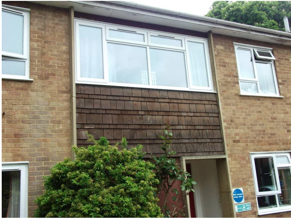
Photograph 03 (Stair well West wing)
